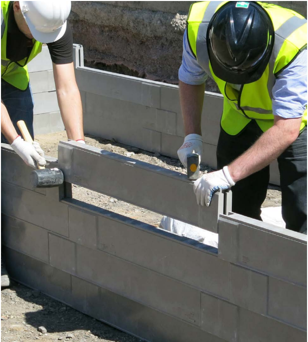
Offsetting joints between sections provide a brickworked design providing strong sidewall performance.
