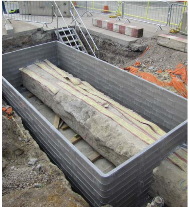
Chamber walls can be built around existing infrastructure.
